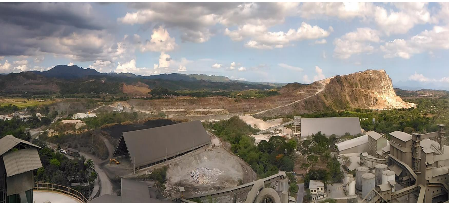
Plate ES1: Panoramic view of the Project Site
