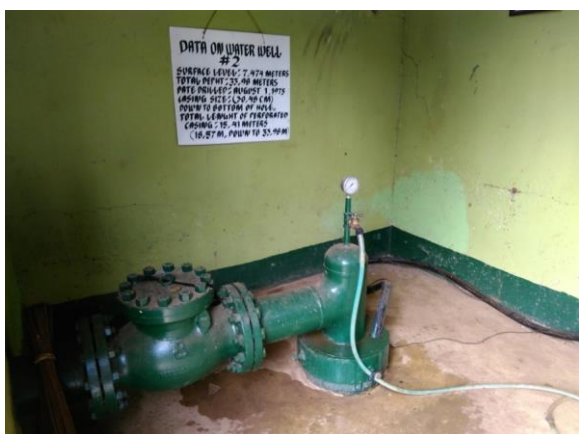
Plate 2.2.16. The well casing and riser pipe of RTNMC Water Well No. 2 (WW2) which is labeled W-6 in the water source location map.
