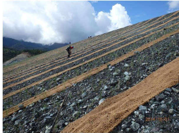
Plate 2.1.3. Slope of TSF2 laid with coconets
