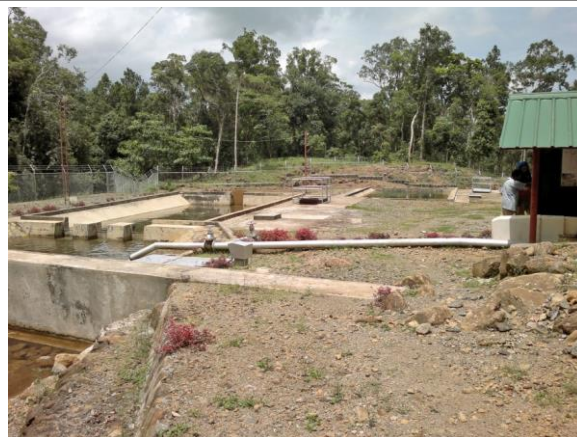
Plate 2.2.13. The raw water treatment facility of the Level III water system fed by Umawi Creek. This facility has several screens and settling ponds to filter and settle suspended solids prior to chlorination.
