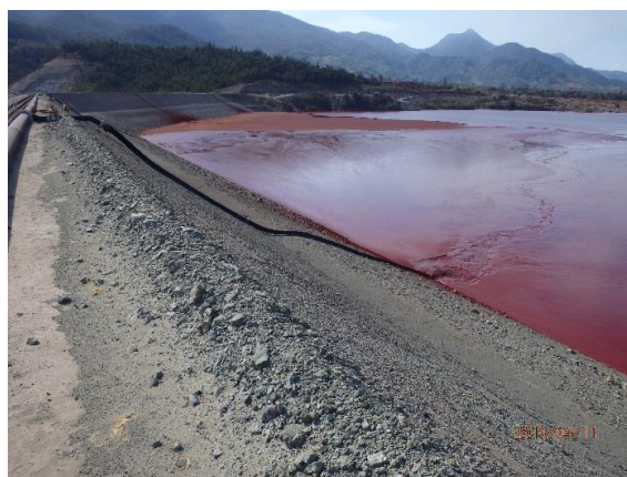
Plate 1.5.6. Tailings discharge to the dam
