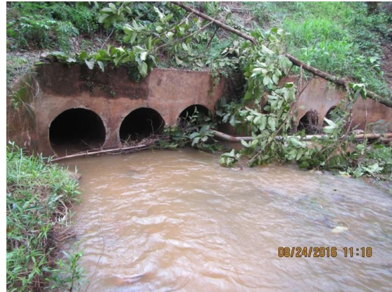
Plate 2.2.4. This diversion canal routes the outflow from Tagpisa Siltation Pond to the Upper Kinurong Siltation Pond which is within the adjacent Tuba River watershed. The water is notably clearer after passing through the Tagpisa Siltation Pond.
