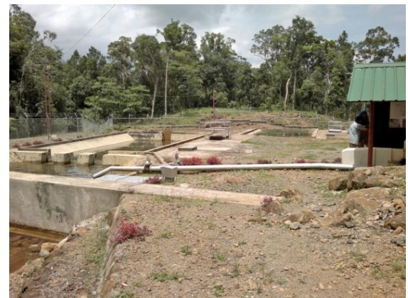
Plate 2.2.11. The raw water treatment facility of the Level 3 water system fed by Umawi Creek. This facility has several screens and settling ponds to filter and settle suspended solids prior to chlorination.
