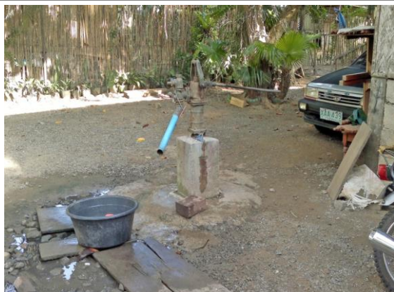
Plate 2.2.5. Shallow cased wells such as this one in Brgy. Ocayan used to be the main source of domestic water in the area surrounding the proposed TSF3.
