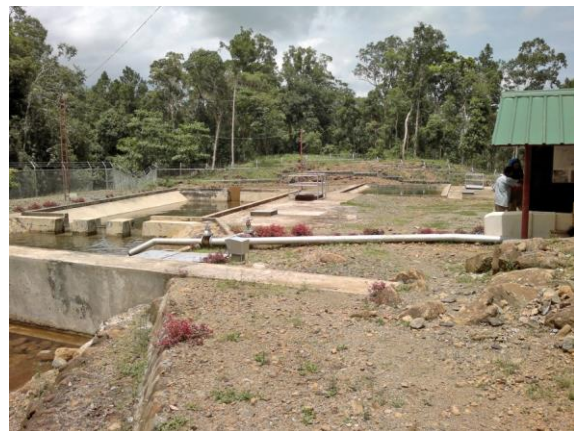
Plate 2.2.9. The raw water treatment facility of the Level 3 water system fed by Umawi Creek. This facility has several screens and settling ponds to filter and settle suspended solids prior to chlorination.
