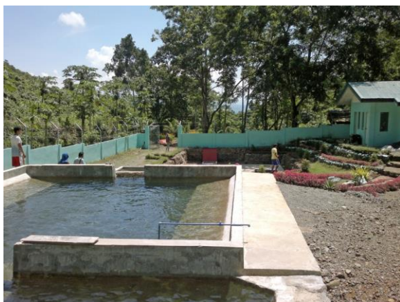
Plate 2.2.14. A series of screens and settling ponds at the raw water treatment facility beside Baracbaracan Creek filter the water of the Level II before it is chlorinated and piped to the users.
