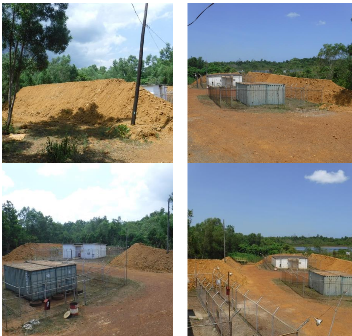
Plate 1.5.13. Constructed berm at the Magazine area
