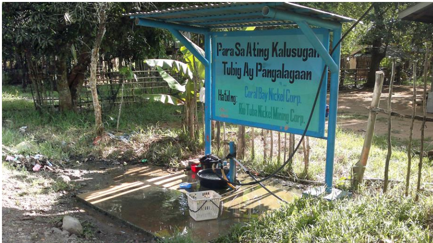
Plate 2.2.5. An outlet of the Level II water system along the provincial highway at Sitio Bicol Village, Bgy. Sandoval. Some hoses were connected to the pipe, allowing the water to reach several homes.
