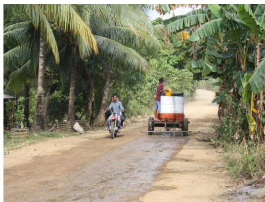
Plate 1.5.11. Water spraying of the hauling road
