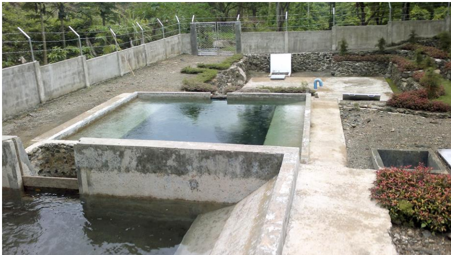
Plate 2.2.4. A series of screens and settling ponds ensures that the water of the Level II water system is clear and free of suspended solids before it is chlorinated and piped to the users.
