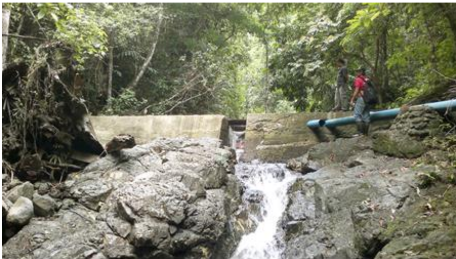
Plate 2.2.3. The dam constructed across the Pasi-Pasi River diverts river water for use in the Level II water system of RTNMC and CBNC.
