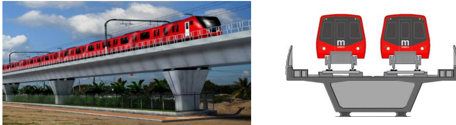
Figure 1.4.1 PC segmental box girder
