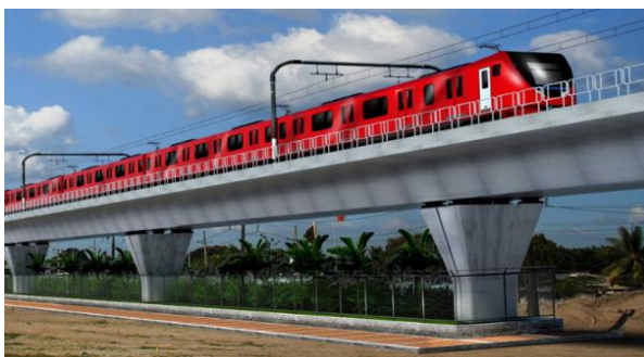
Figure 1.4.1 PC segmental box girder
