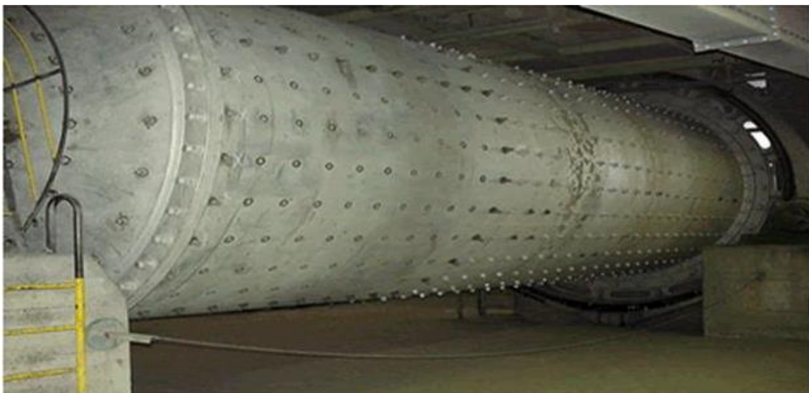
Plate 6: Cement mill being used in cement grinding
