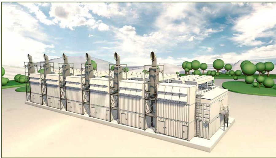
Figure 1-9. Modular Diesel Power Plant
