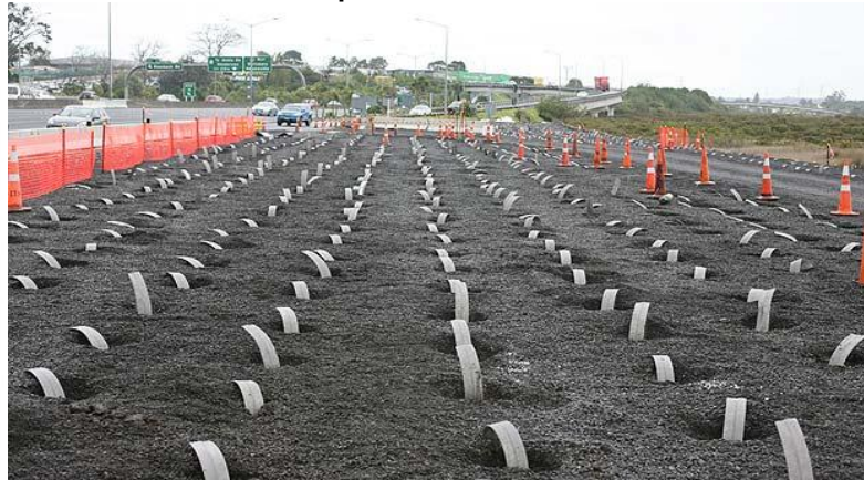
Plate PD-7. Illustration of the Principle of Wick Drains
