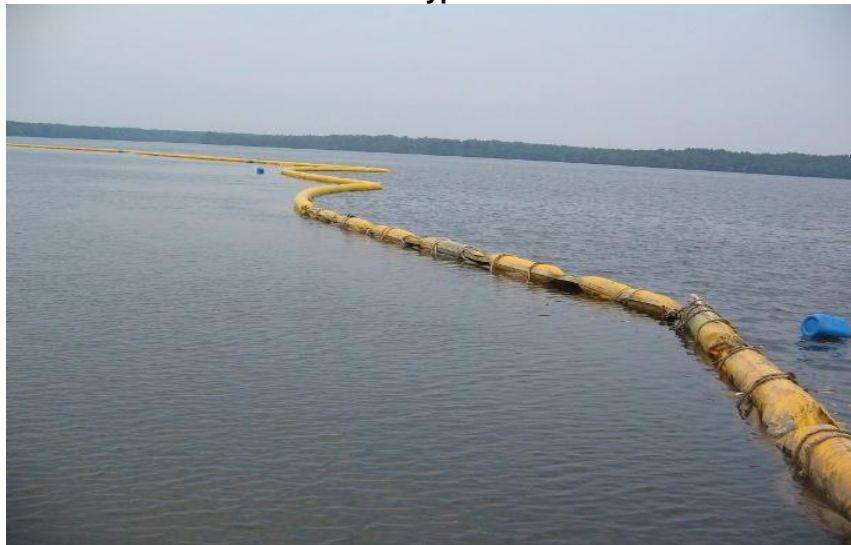
Plate PD-1. Typical Silt Curtain Installation
