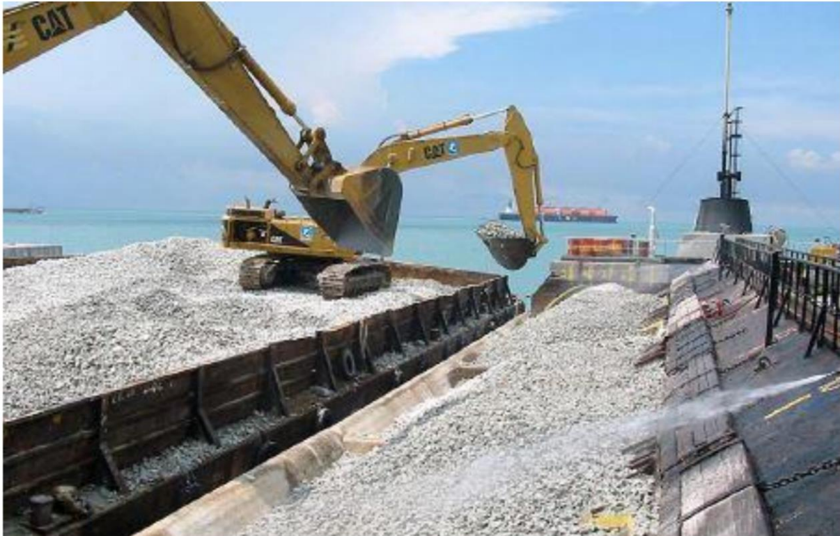
Figure 1-24. Typical excavator unloading the materials from a Hopper Barge (Source: IADC, 2014)
