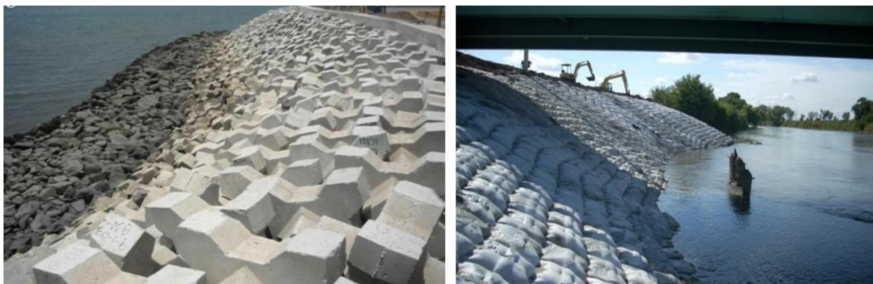
Figure 1-13. Examples of sloping revetment (left: concrete blocks, right: concrete mattress)
