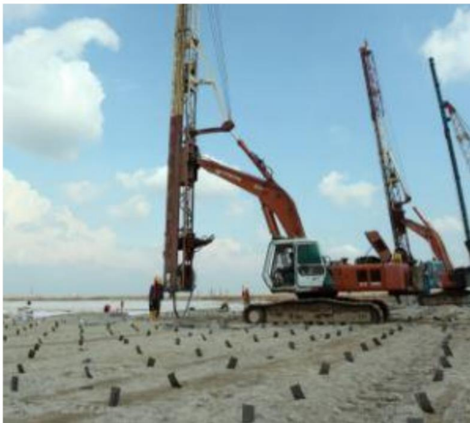
Figure 1-15. Installation of PVDs.
