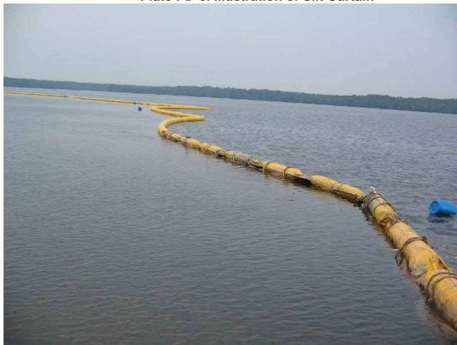
Plate PD-6. Illustration of Silt Curtain
