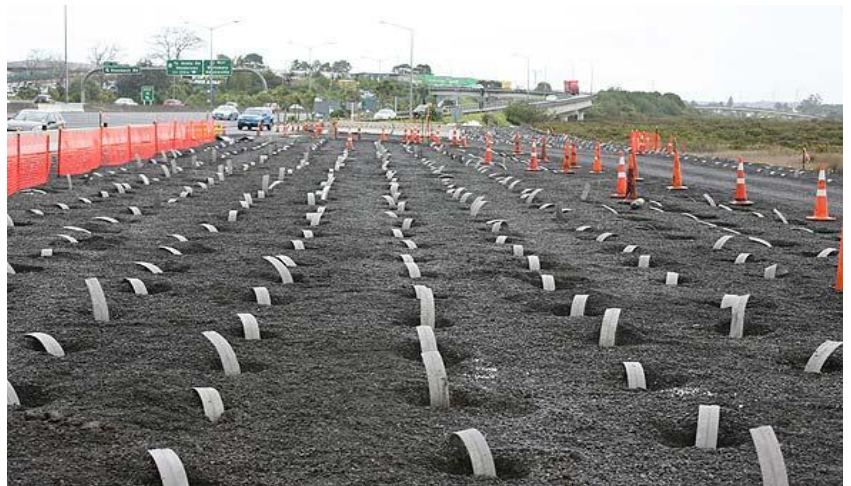
Plate PD-3. Illustration of the Principle of Wick Drains
