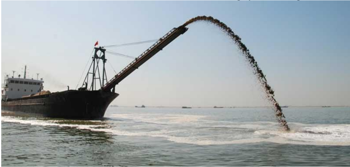
Plate PD-7. Illustration of Sand Filling by Rainbowing
