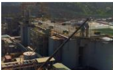
The process plant's CIL tanks (PGPRC photo).
