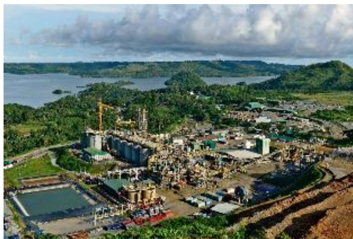
PGPRC's processing plant complex with the CIL tanks, power plant stacks, decant water treatment plant, and process water pond as the prominent features. FRC's heavy equipment workshop is visible right side of the complex. Port Barrera is seen at the background (PGPRC photo).
