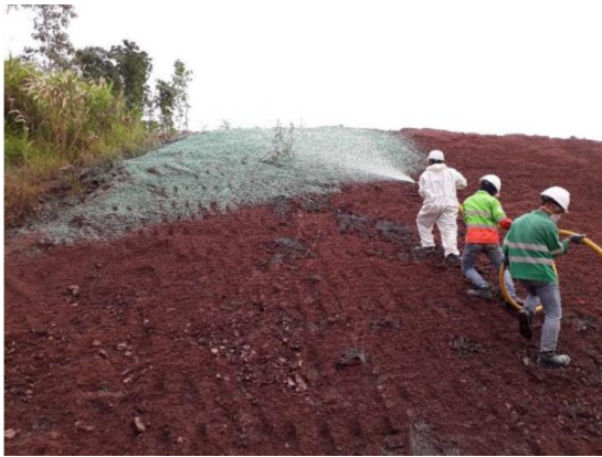
Photo 6-10: MacFlex application on Trial Slopes
