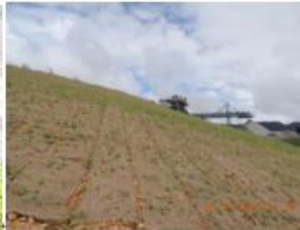
Photo 6-7: Cocomatting and revegetation at ROM ringroad
