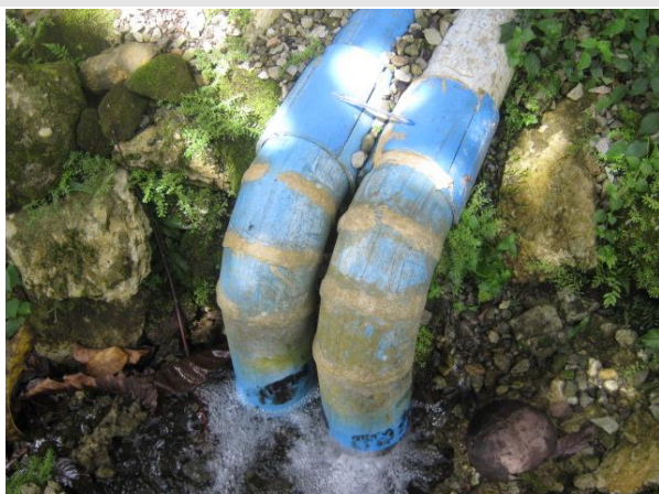
Plate 2.2.1-12 Discharge Pipes from Intake Box
