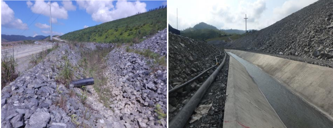
Photo 6-1: Rock lining and rock surfacing
