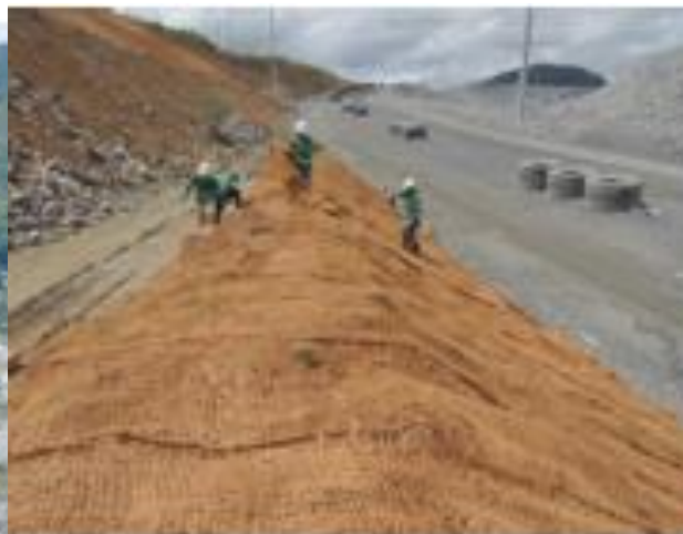
Photo 6-9: Cocomatting at lower Boya dump area
