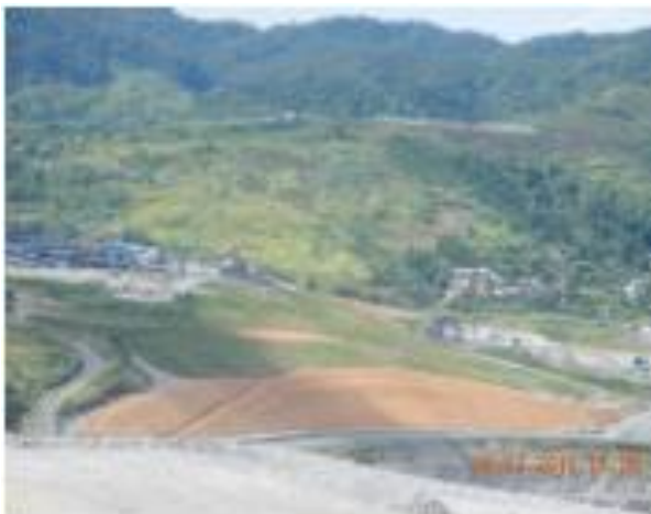
Photo 6-8: Cocomatting and revegetation at ROM northwall
