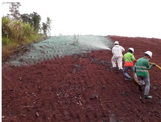
Photo 6-10: MacFlex application on Trial Slopes
