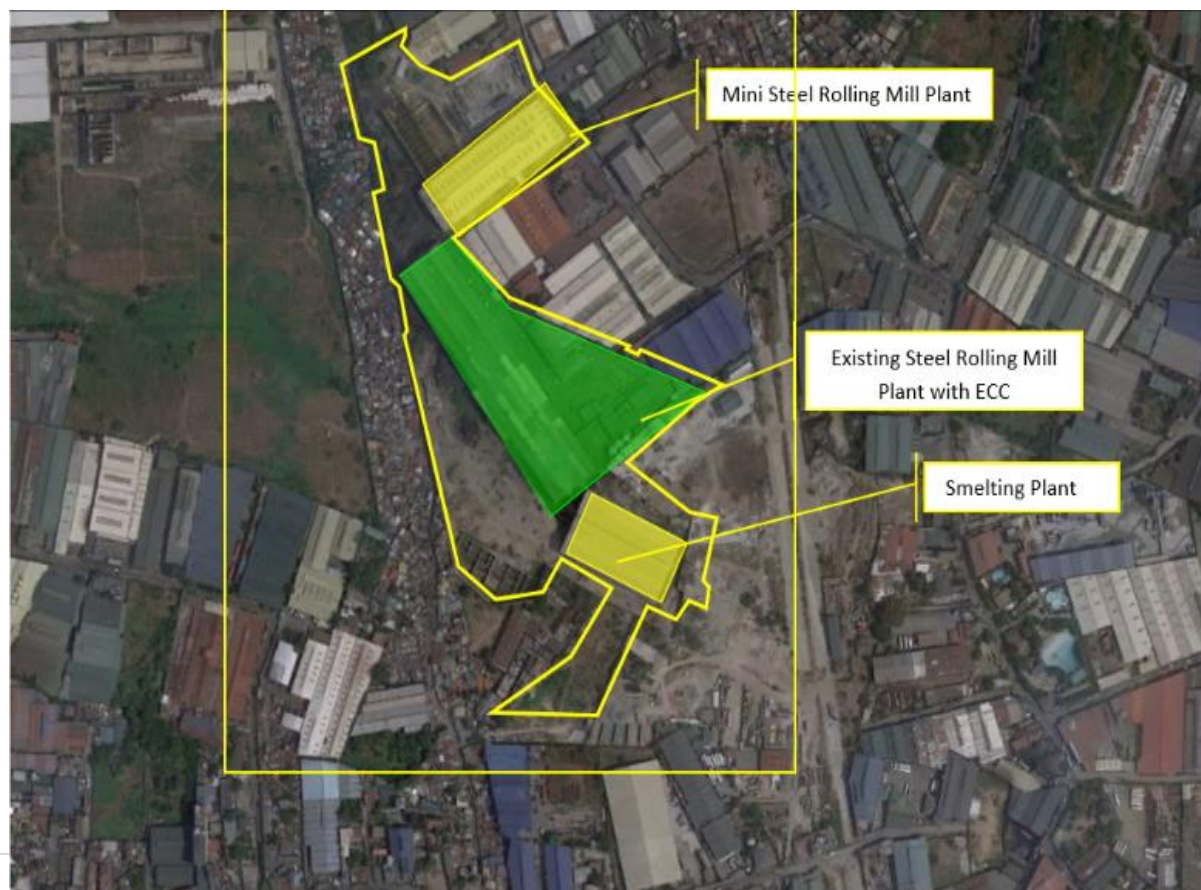
Figure 6: Satellite View of the Existing Steel Rolling Mill and the Newly Constructed Smelting Plant and Mini Rolling Mill
