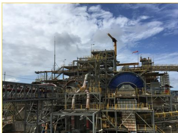
The existing mills in the Processing Plant. Arrangement from right to left: SAG Mill, BM No. 1, BM No. 2
