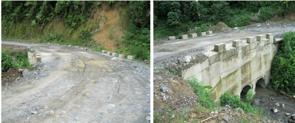
Two-barrel concrete spillway constructed January 2013 At Km. 28, Hinalaan, Kalamansig. S.K
