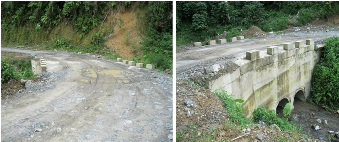
Two-barrel concrete spillway constructed January 2013 At Km. 28, Hinalaan, Kalamansig. S.K
