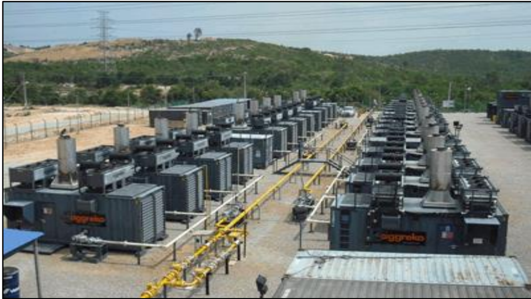
Figure 8. Modular Diesel Power Plant Set-Up
