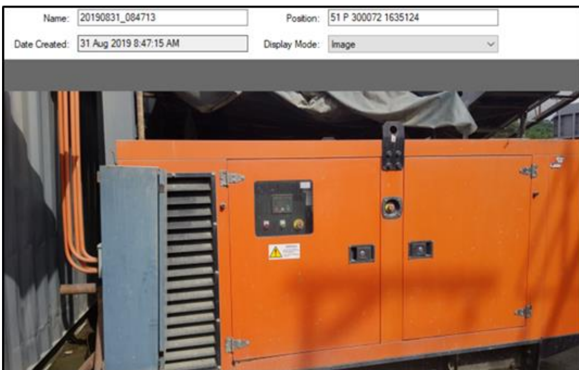
Photo 25. Generator set (600 kVA) used for welding machines
