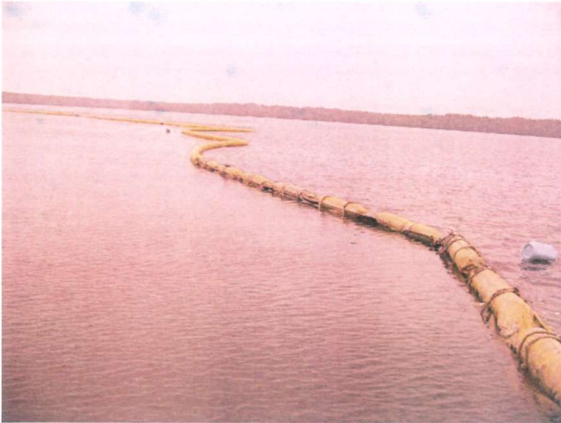
Plate A.2 Illustration of Silt Curtain
