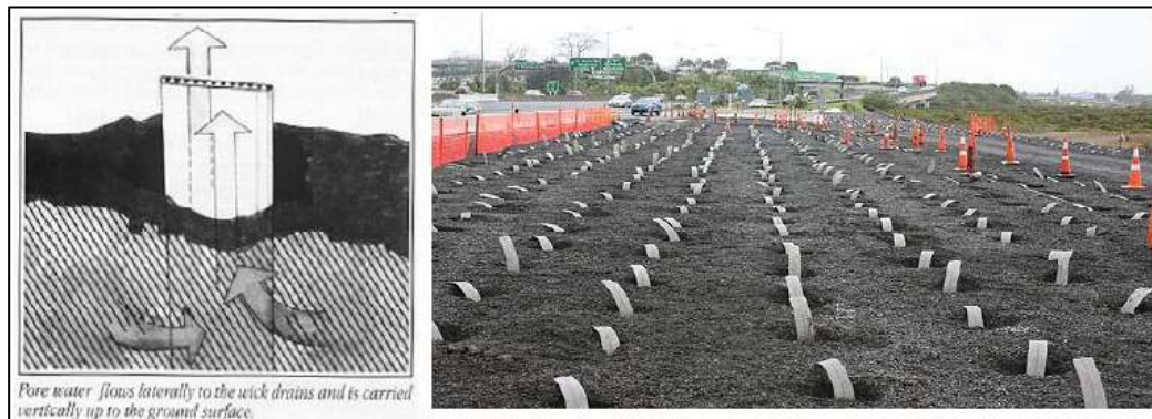
Plate 1-13. Illustration of the Principle of Wick Drains
