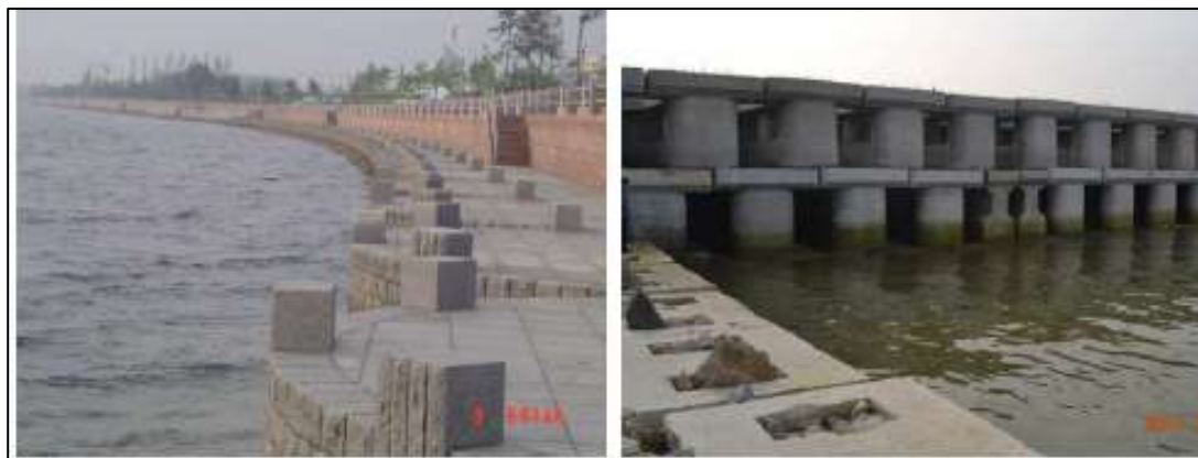
Plate 1-1. Vertical Gravity – type Dike
