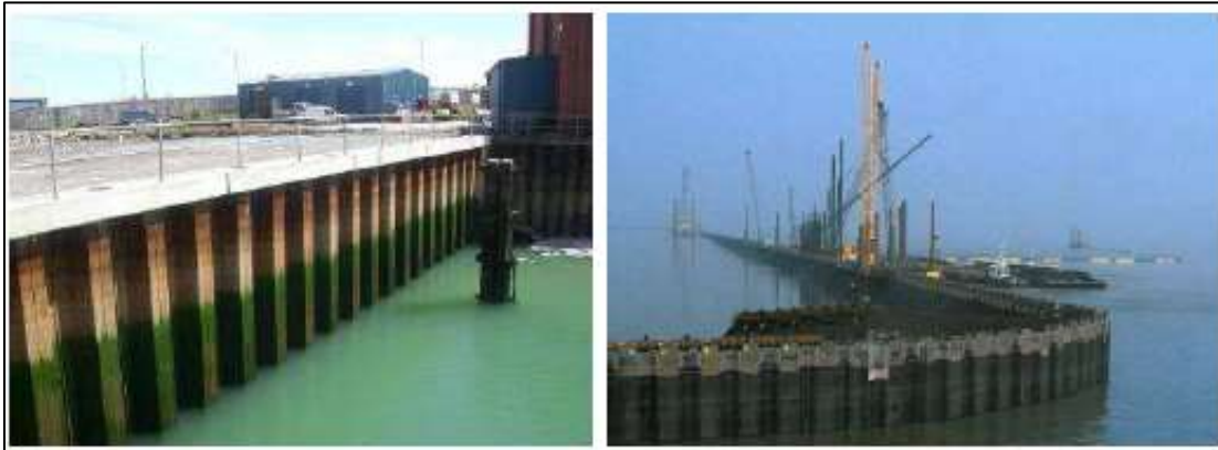
Plate 1-2. Vertical Pile Foundation Dike
