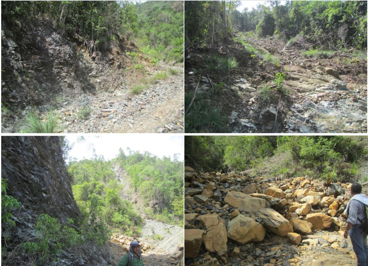
Figure 2.1-30. Photos of slopes and landslides along the access road within the MPSA area. Clockwise from top: highly fractured rocks prone to rockfall along the road; scar of debris flow track; dominantly large boulders debris flow deposit in one of the stream crossing; and landslide originating from the ridge.
