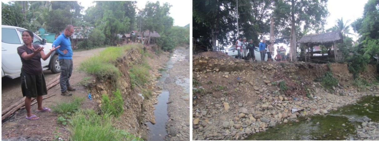
Figure 2.1-43. Riverbank erosion in Sitio Trinidad (Purok 8) in Brgy. Maputi. Two houses were carried by flood in October 2015 due to scouring. The flood depth along the road is around ankle deep but in the channel, flood depth is about 5 m.
