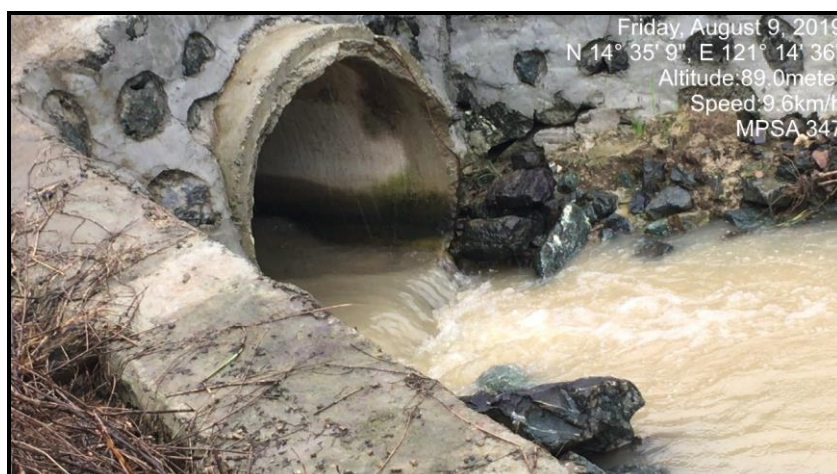
Photo 2aaaa. Existing RCP Pipe as drainage connected from the Culvert along Pantay-Buhangin Road, run-off is served as the irrigation (After the rain scenario)
