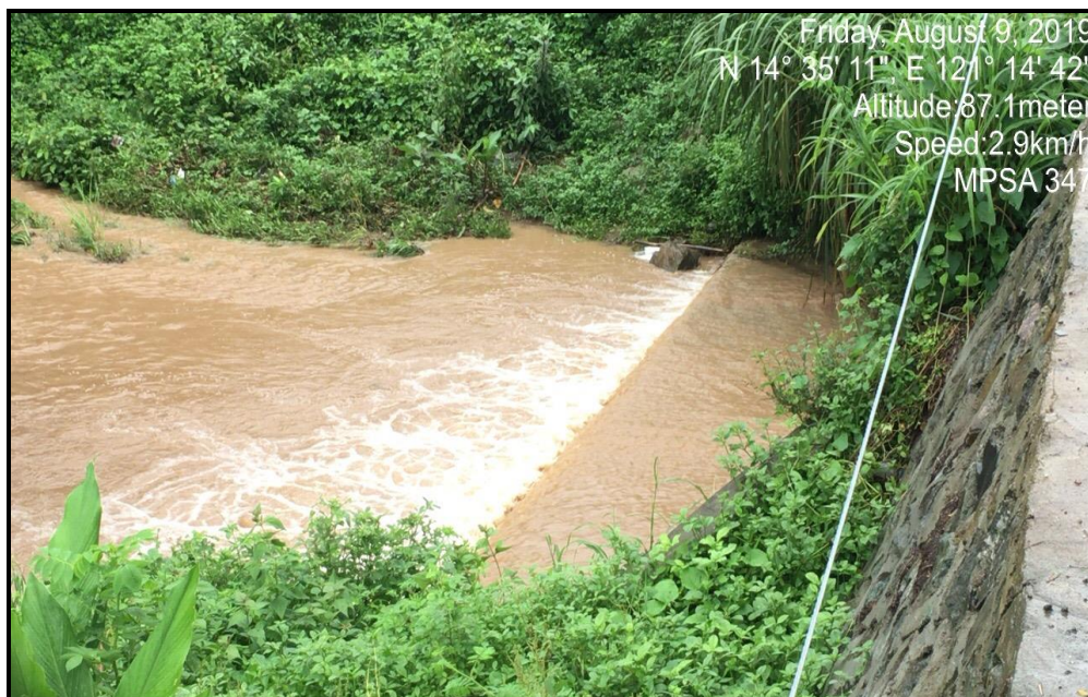
Photo 2yyy. Box Culvert serves as drainage outfall along Pantay-Buhangin Road, rainwater is captured at the lowest elevation (After the rain scenario)
