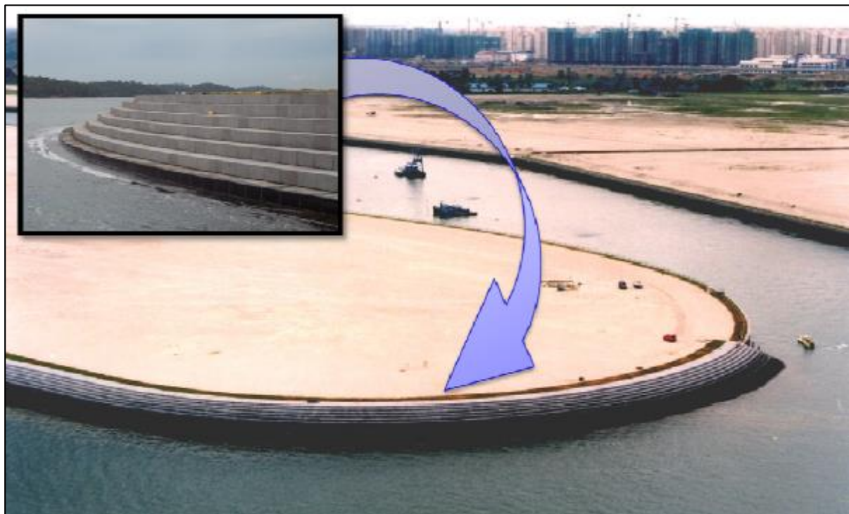
Figure 1-5 Stepped Sloping Seawall used in the Northeastern Coast Reclamation in Singapore
