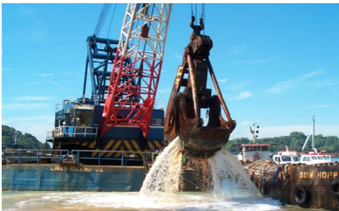
Figure 1-10 Dredging of the Trench
