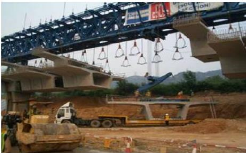
Figure 1.17 Gantry Construction of Viaduct, Hong Kong
