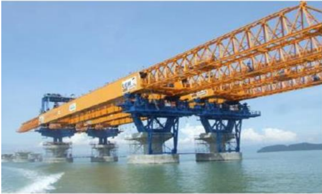
Figure 1.16 Gantry Construction of Penang Second Bridge, Malaysia
