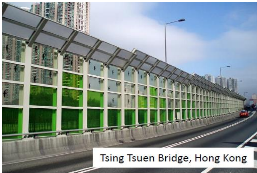
Figure 1.20 Illustration of Noise Barrier Installed in Tsing Tsuen Bridge, Hong Kong
