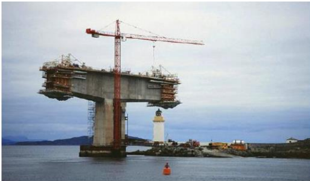
Figure 1.13 Typical In-situ balanced cantilever construction of the Skye Bridge, Scotland
