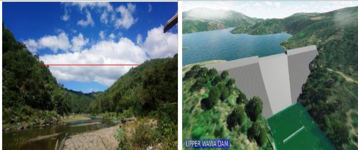
Figure EL-31. Left photo shows existing site condition facing downstream with the dam axis represented by the red line vis-à-vis the perspective view of proposed Upper Wawa Dam facing upstream.
