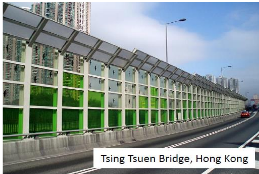
Figure 1.49 Illustration of Noise Barrier Installed in Tsing Tsuen Bridge, Hong Kong
