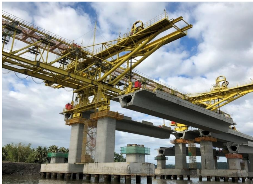
Figure 1.44 Full Span Erection of Marine Viaducts, Brunei Temburong Bridge
