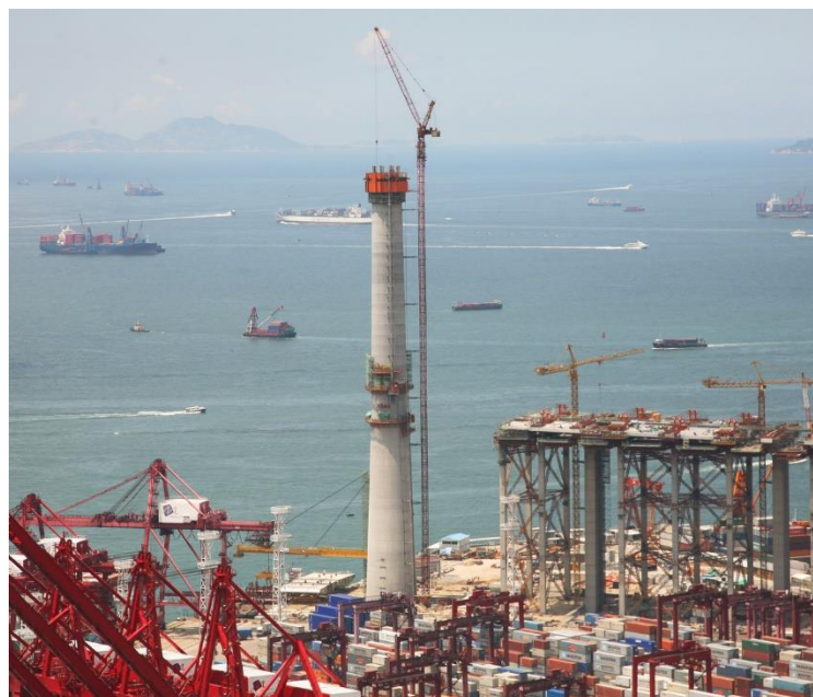
Figure 1.39 Moving Formwork Construction
