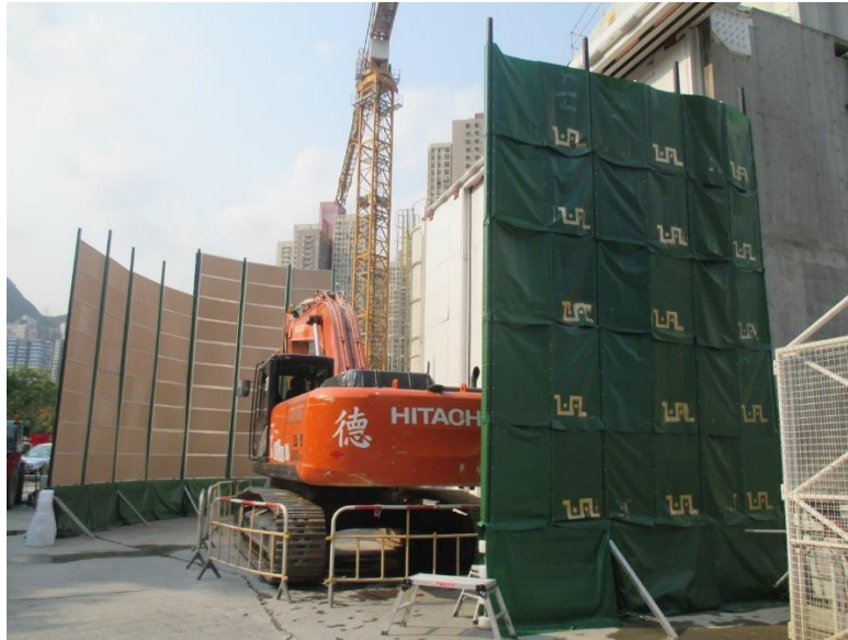
Figure 1.37 Movable noise barrier next to an excavator
