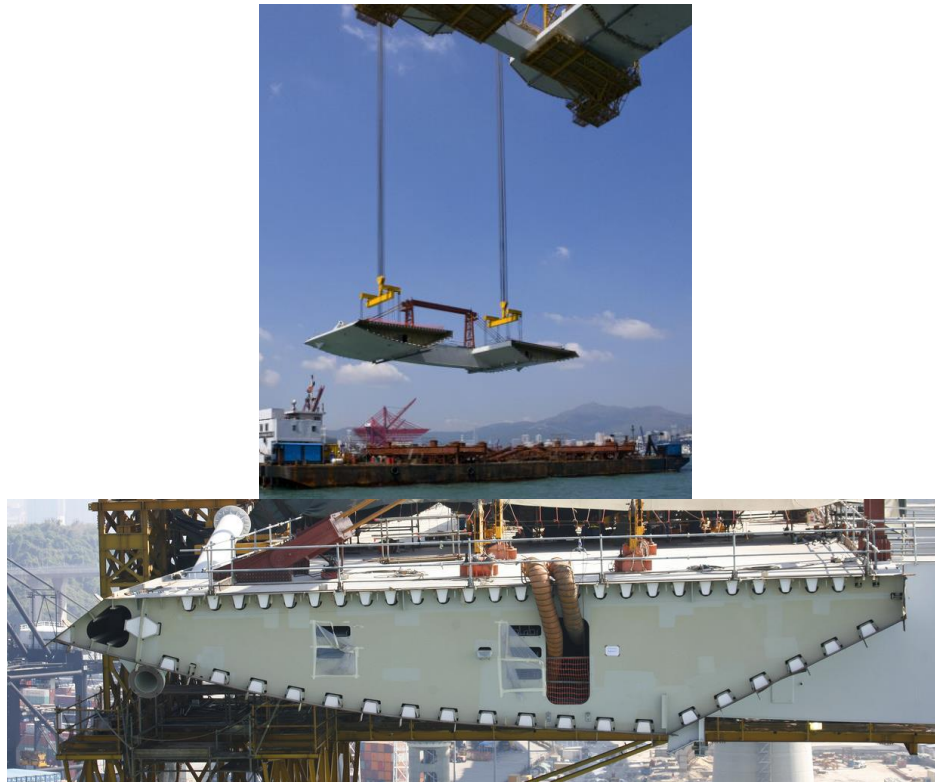
Figure 1.40 Split steel boxes during deck erection phase of Stonecutters Bridge
