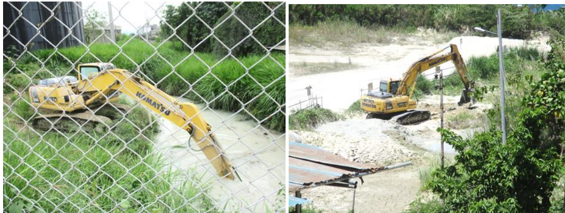
Desilting of Settling Pond No. 1 Stage 1 (left) and Settling Pond No. 4 (right)
