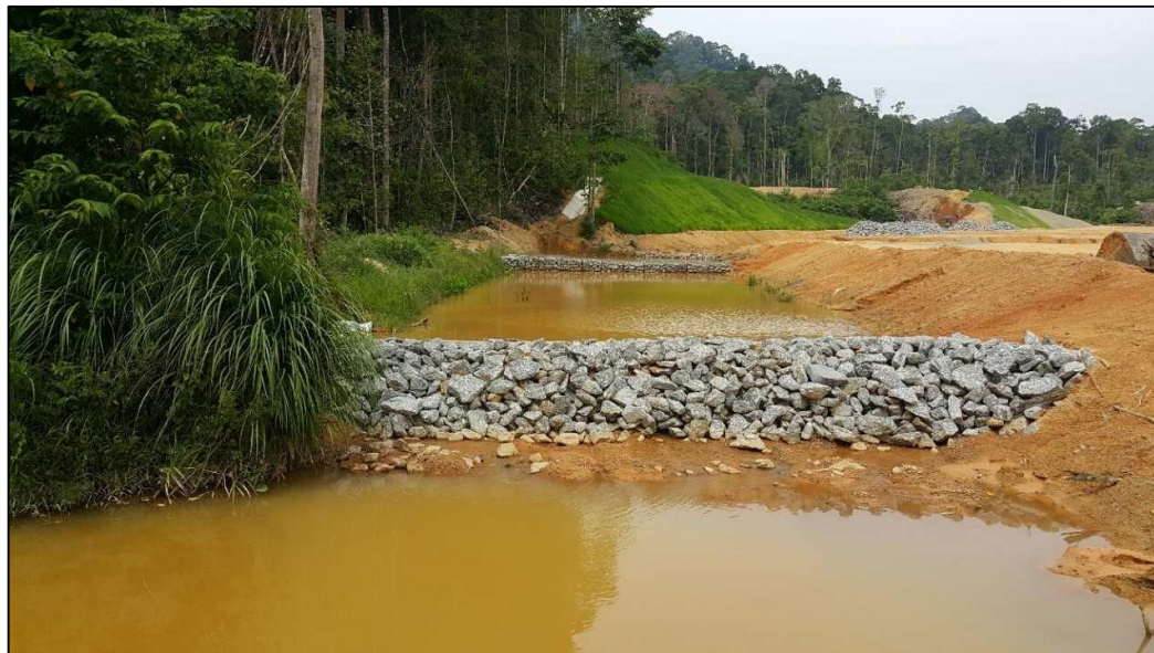
Figure 3. 2 Sample of Continuing Series of Settling Ponds
