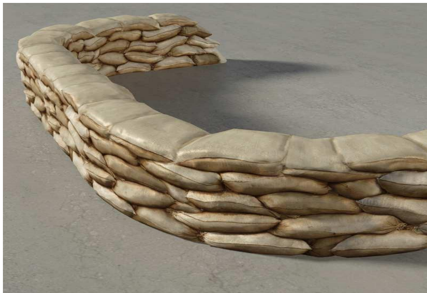
Figure 3. 3 Sandbag Lay-out to control Sediment Flow
