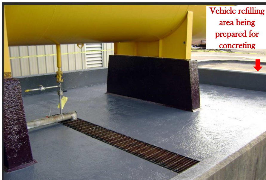
Figure 3. 7 Example of Concrete Flooring with Lip in Fuel Storage Depot
