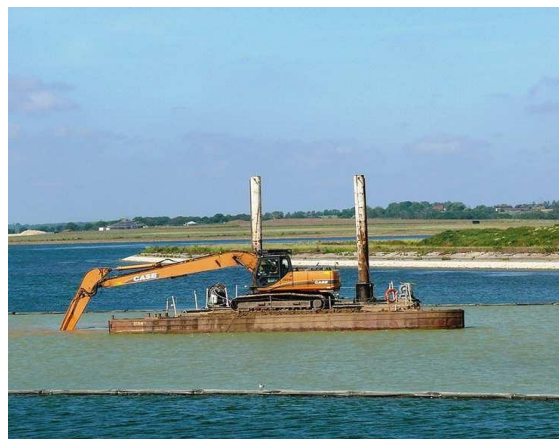
Figure 3. 6 Silt Boom Enclosing an Area with Seabed Disturbance
