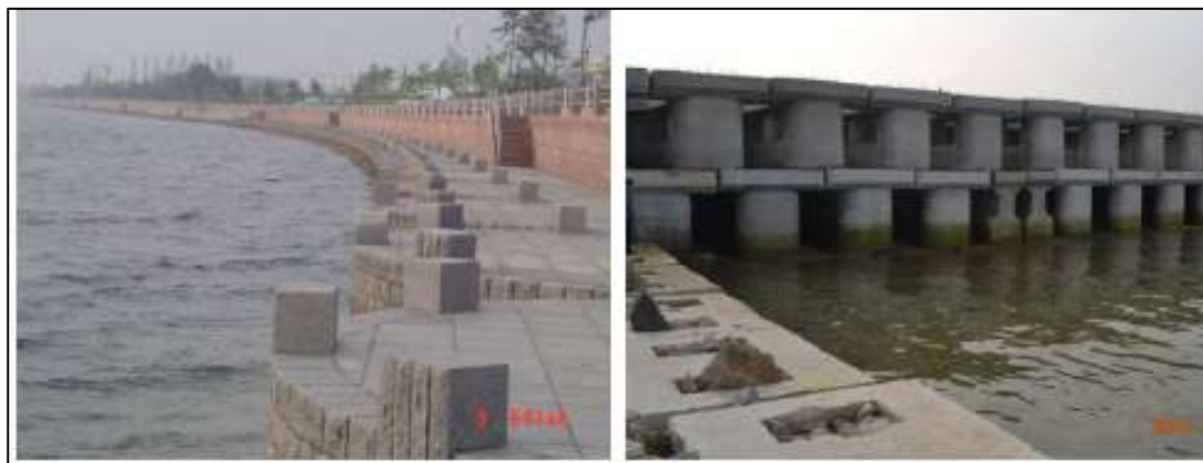
Plate 1-1. Vertical Gravity – type Dike
