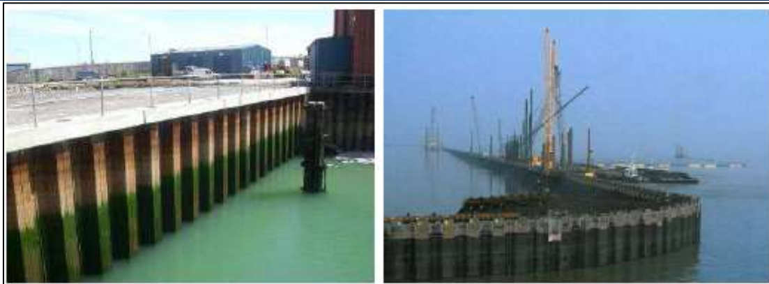
Plate 1-2. Vertical Pile Foundation Dike
