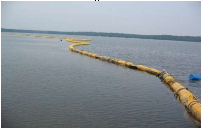
Plate 1-10. Typical Silt Curtain Installation
