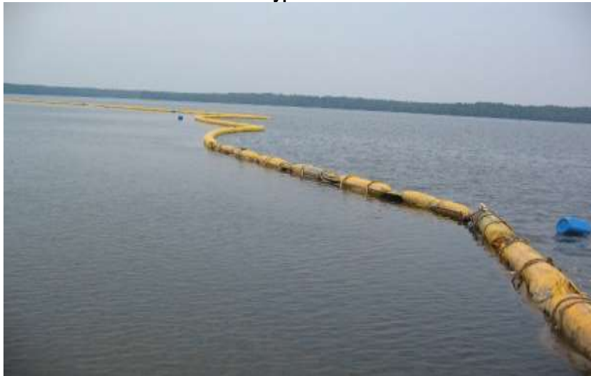
Plate 1-9. Typical Silt Curtain Installation
