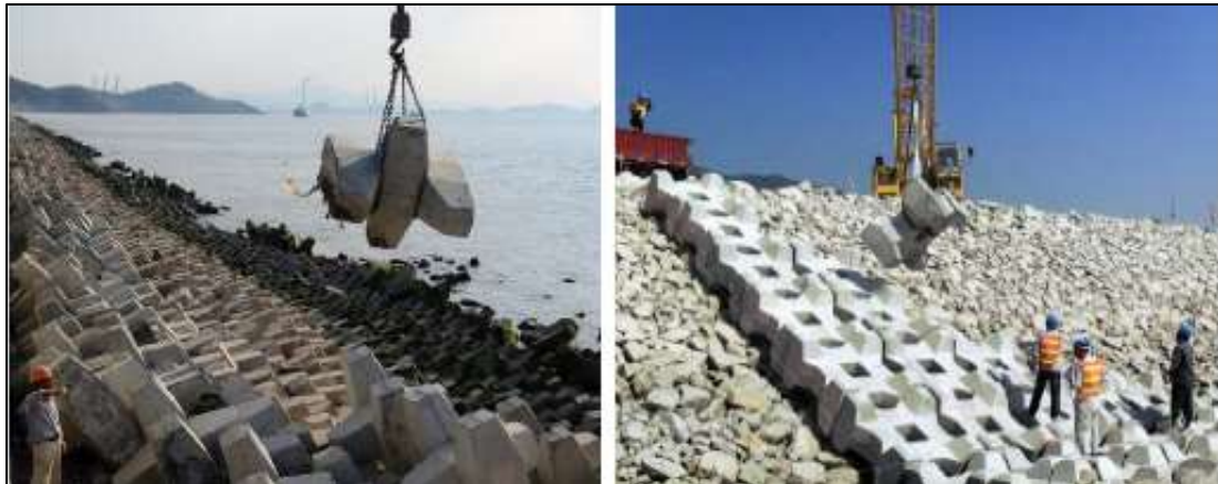
Plate 1-6. Artificial Block Armor
