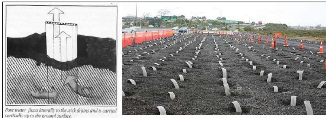
Plate 1-14. Illustration of the Principle of Wick Drains
