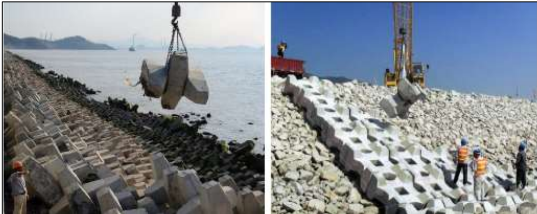
Plate 1-6. Artificial Block Armor
