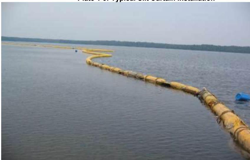
Plate 1-9. Typical Silt Curtain Installation
