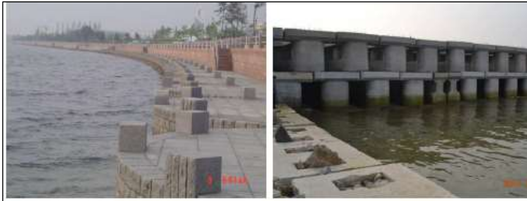
Plate 1-1. Vertical Gravity – type Dike
