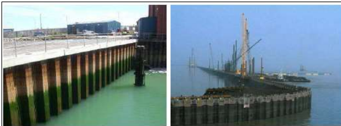
Plate 1-2. Vertical Pile Foundation Dike
