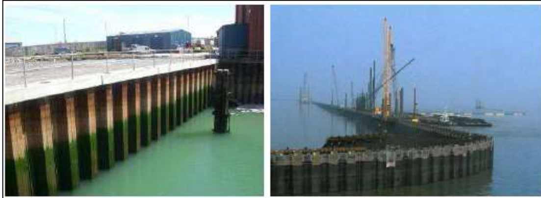
Plate 1-2. Vertical Pile Foundation Dike
