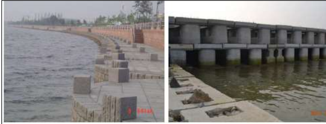
Plate 1-1. Vertical Gravity – type Dike
