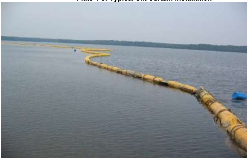
Plate 1-9. Typical Silt Curtain Installation
