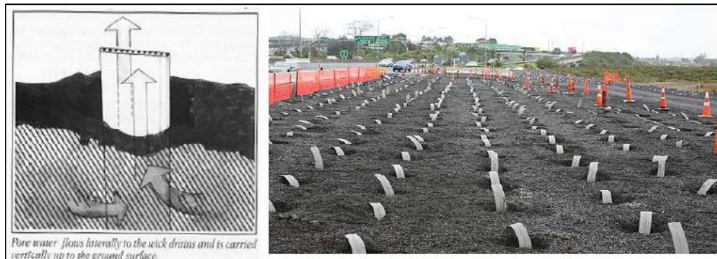
Plate 1-13. Illustration of the Principle of Wick Drains
