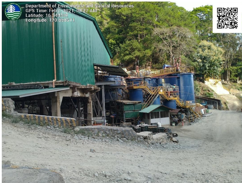
Figure 2-15: Existing 200TPD CIP Plant Set-up.
