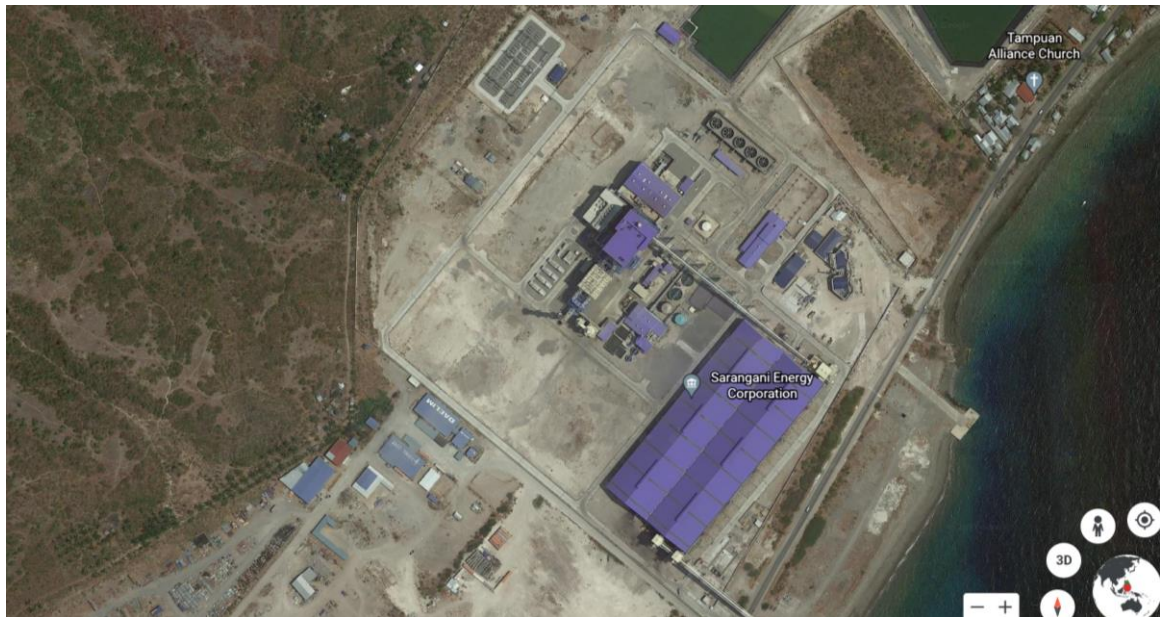
Adjacent Energy Plant of the Proposed Project
