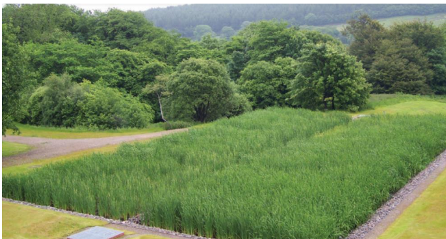
FIGURE 1-14. REED BEDS USED FOR WASTEWATER TREATMENT
