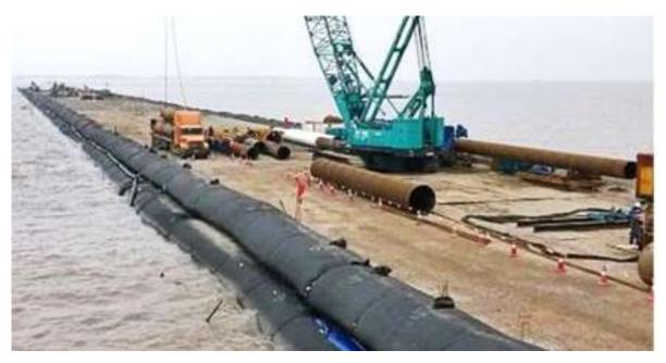
Figure 1-96 Placement of Geotextile Tube
