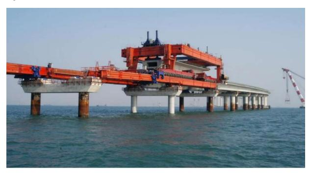
Figure 1-85 Pile Bent Support of Incheon Bridge Viaduct, Korea
