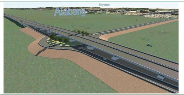
Grade-separated roundabout is type of interchange connecting between a highway and minor roads. The slip roads to and from the highway converge at a single roundabout, which is grade-separated from the mainline with bridges. The roundabout allows for multiple direction of connections with minor roads in a one direction of flow around a central island. This type of interchange allows for free flow of traffic to be maintained along the highway mainline.
