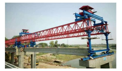
Figure 1-86 Precast Beams Erected by Back Feed Launching Gantry
