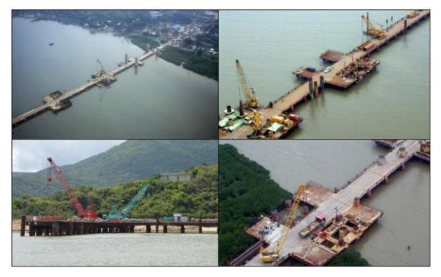
Figure 1-83 Temporary Steel Deck Access and Working Platform for Piling Machines
