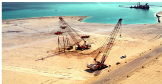
VIBRO COMPACTION
