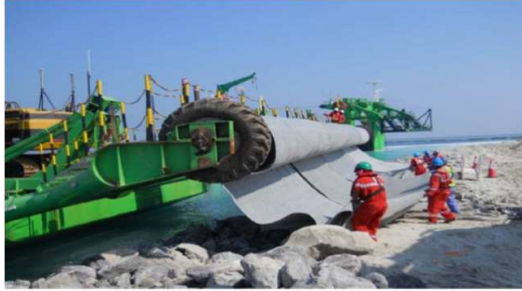
INSTALLATION OF GEOTEXTILE MEMBRANES
