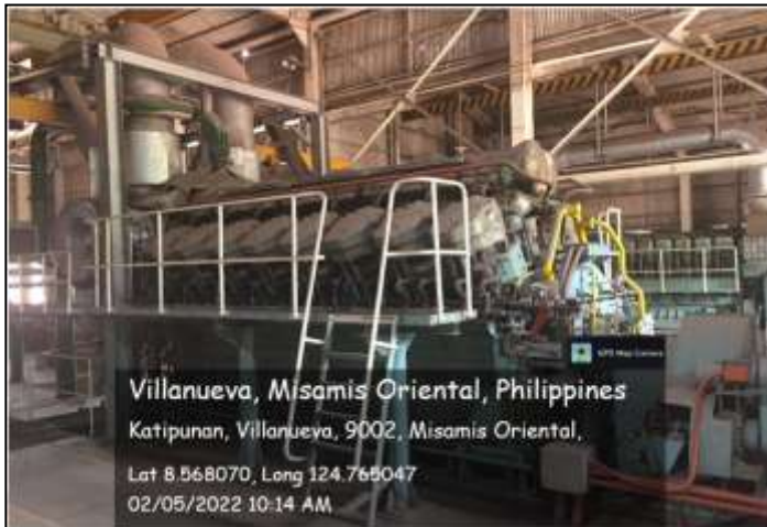
5.5 MW Diesel Generator
