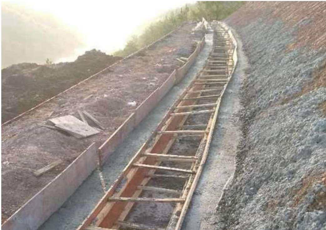
Figure 1.10: Detail of cut off ditch
