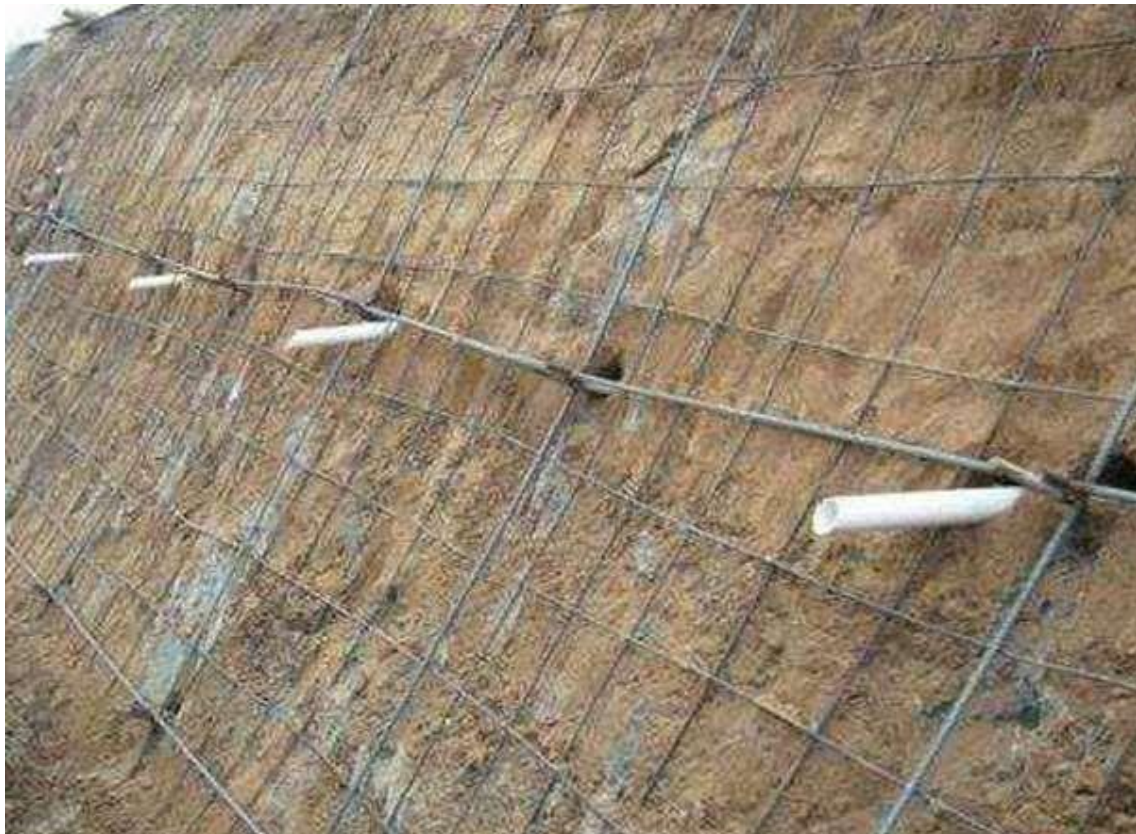
Figure 1.9: Anchor bar with wire mesh and PVC horizontal drains
